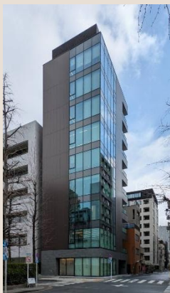
DEAR LIFE Nihonbashi-Hamacho Building
